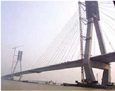
(a) Cable-stayed portion
